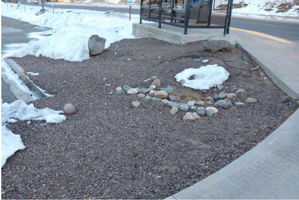
Figure 1-8: Culvert outlet in NAU parking lot 46
