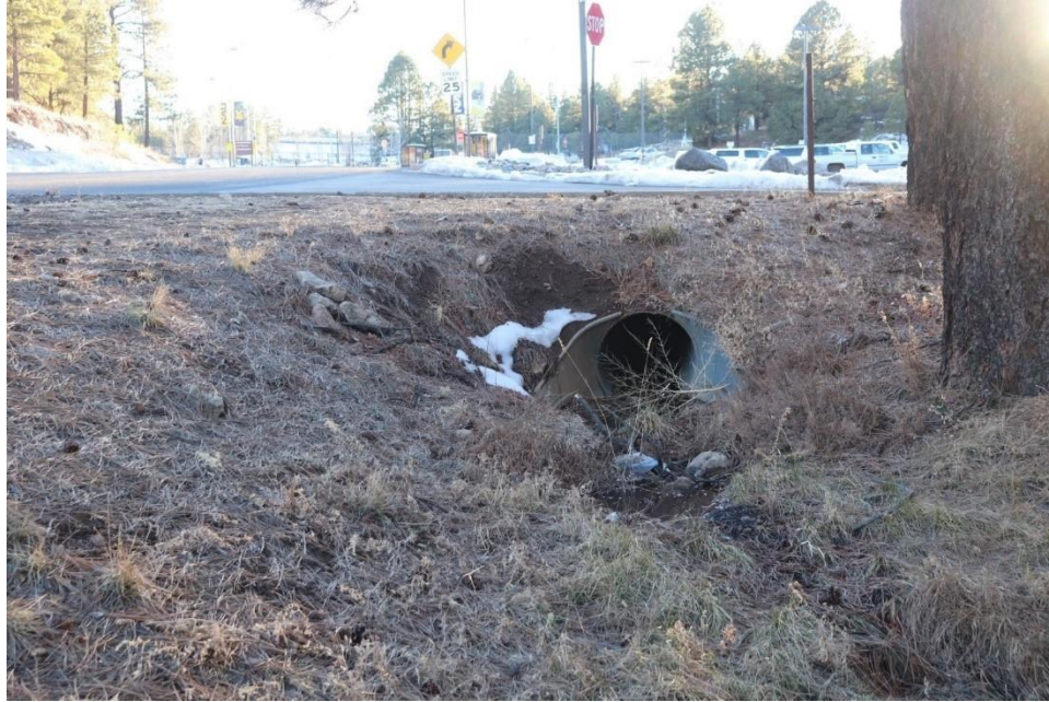
Figure 1-10: Culvert drainage outlet near Rolle Activity Center
